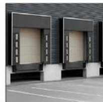
I CONCRETE DOCK WALL & DOCK SEAL
