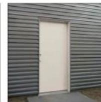
K POWDER COATED STEEL DOORSET COLOUR TO MATCH CLADDING, SUBJECT TO LOCATION
